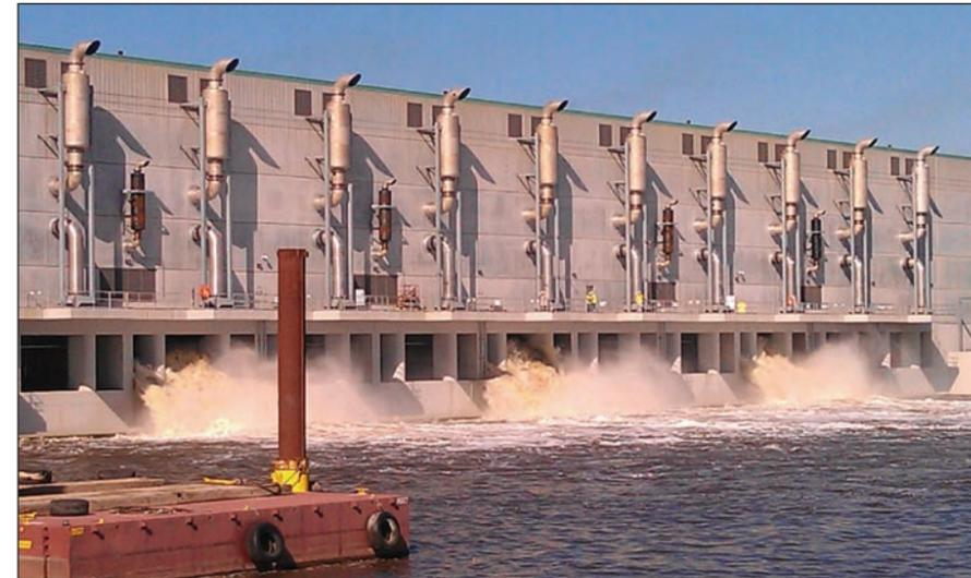
The world's largest drainage pump station keeps water flowing out of town, even when the nation's largest sector gate closes the waterway. PHOTO COURTESY OF WENDI GOLDSMITH
